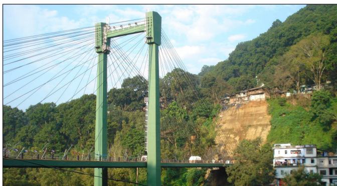
Figure 2. Landslide near the cable-stayed bridge at Nayabazar (South Sikkim District) restricted the use of the bridge for relief work after the earthquake (photo: C.V.R. Murty).
