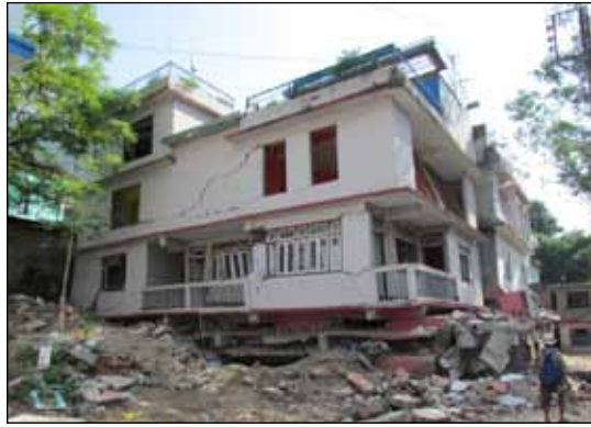
Figure 5. Pancaking of three stories in five-story house in Jorethang, South Sikkim (photo: A. Sheth).
