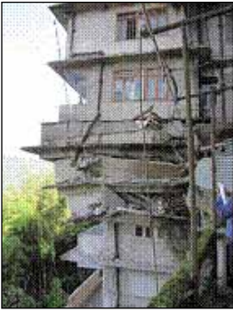
Figure 4. Pancaking of middle two stories in a nine-story building at Gangtok, East Sikkim (photo: D. Rai).
