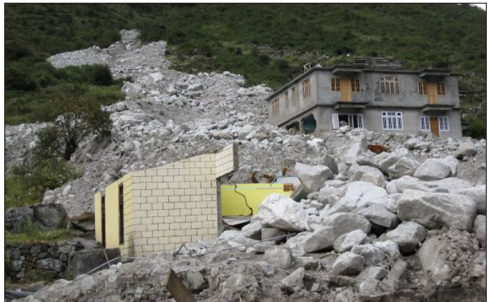
Figure 3. Damage due to rockslide and mudslide at Lachung (photo: D. Rai).
