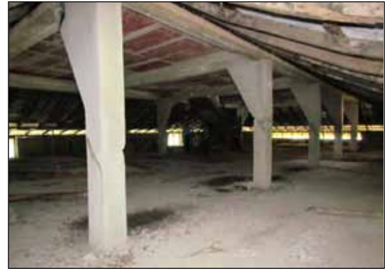
Figure 6. All columns supporting roof of Phudong Monastery, North Sikkim, failed. (photo: A. Sheth).
